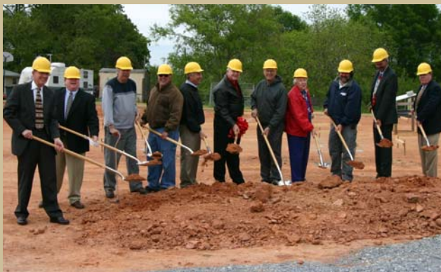
Groundbreaking for Americ-Inn of Boiling Springs (428 East College Avenue) on April 26.
